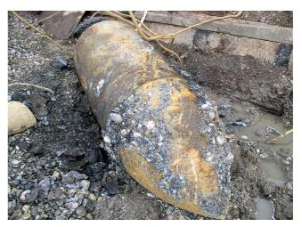
The magnetometer cone clears the way for piling, excavation and tunnelling by confirming a site is safe from unexploded ordnance. Obstacles can be avoided by using the information to modify pile location plans or to conduct a bomb clearance programme if necessary. It is vital for the redevelopment of locations where ordnance or buried obstructions may pose a special risk - such as sites that were subjected to wartime bombing, and former military ranges.
